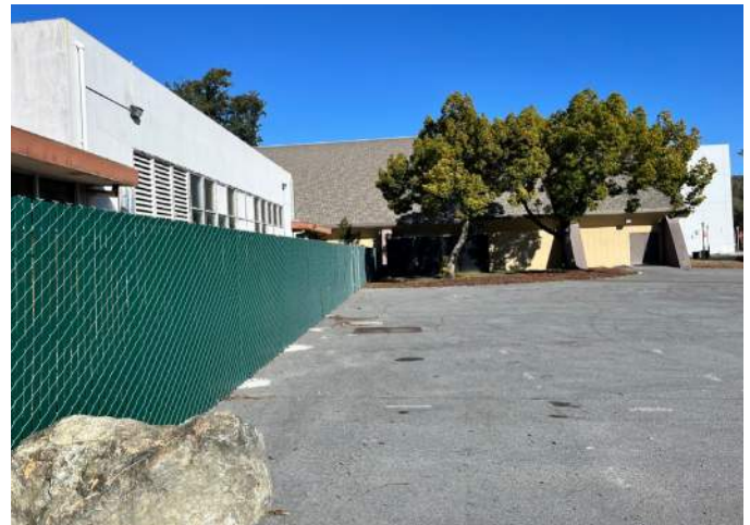
Photo: The locker rooms are scheduled to be demolished. The “smile” path could then be completed.
