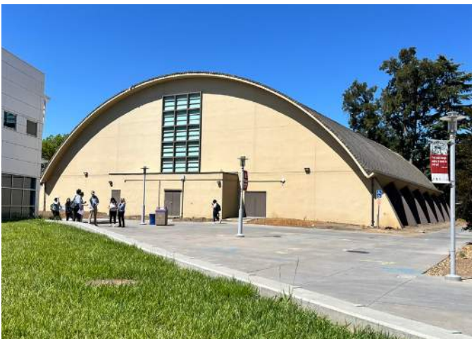
Photo: The arched ends of the gym are an opportunity for more placemaking and activation.
