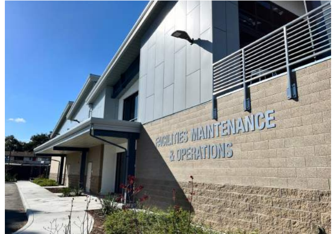
Photo: The new Facilities Maintenance and Operations Building was completed as part of the last SJCC FMP.
