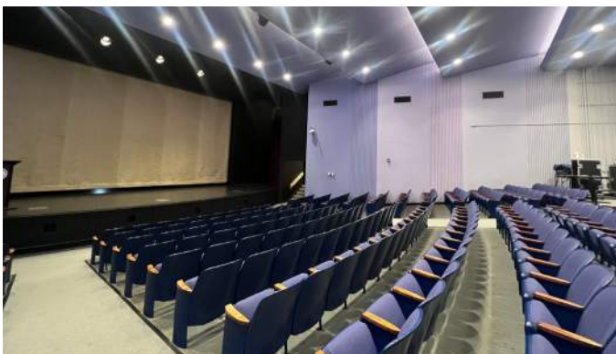
Photo: Even though there have been recent renovations, the slope of the floor and audience seating area are not in compliance.
