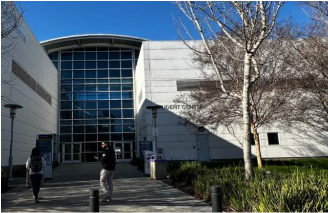
Photo: Building signage is hard to read and there are many legacy types of signage.
