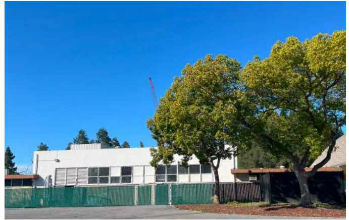
Photo: After you pass through the SC, the soon-to-be-demolished locker rooms are the first thing you see.
