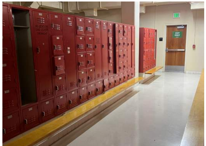
Photo: The locker rooms are dark and have old plumbing fixtures.
