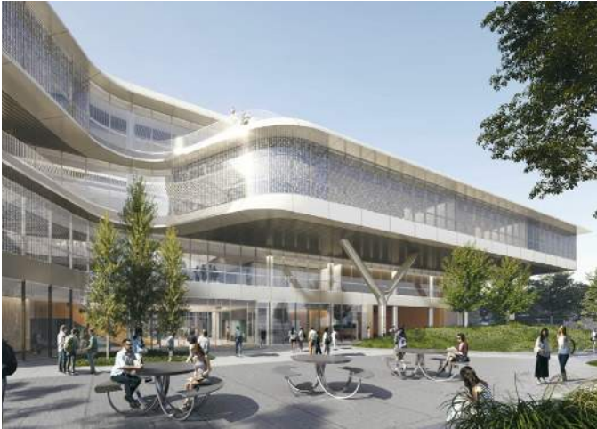
Photo: The Career Education Complex is under construction.
