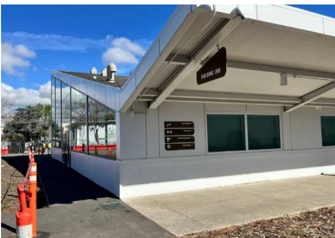
Photo: The 200 Building was renovated.
