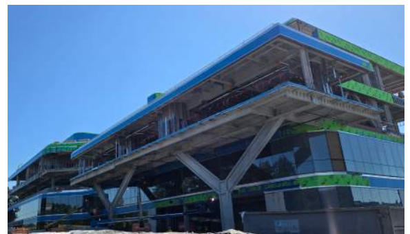
Photo: The Career Education Complex, under construction at San José City College, was funded by Measure X.
