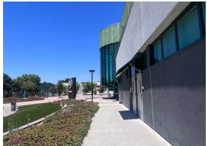
Photo: There are small awnings over the doors at the ground floor, but more covering to protect from the elements is desired.
