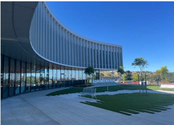
Photo: The new Student Services and Administration Building
