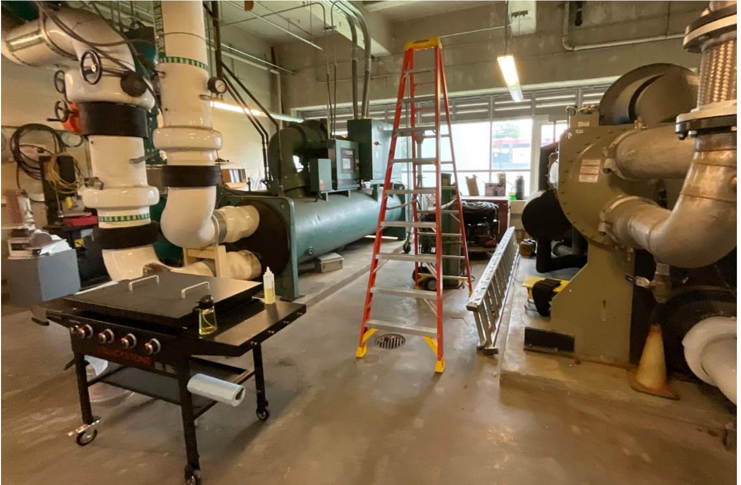
Photo: The access to rooftop equipment is poor. Most of the access is either via the use of a cat ladder or no access is provided, and a ladder is needed to access roof hatches and roof-top equipment.
