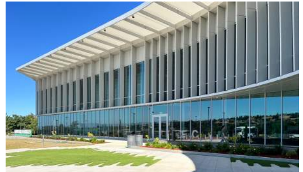
Photo: The new Student Services and Administration Building at Evergreen Valley College that opened in fall 2024 was one of several new buildings that resulted from the previous Facilities Master Plan Update. The SJECCD FMP update for 2027-2037 will include a new list of district-wide improvements.
