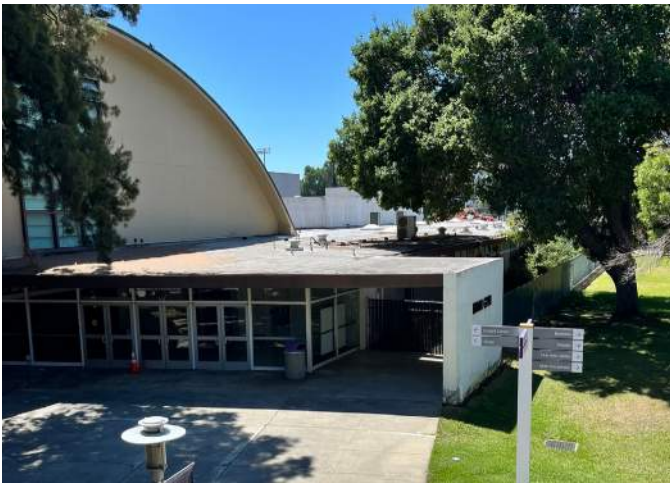
Photo: The lobby of the gym is scheduled to be demolished. This is one of the first views from the main drop-off.
