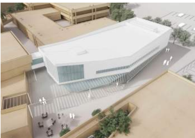
Photo: The Sequoia Nursing addition (under construction fall 2024)
